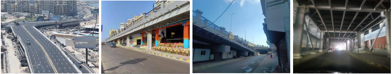
Figure 10. Lost urban spaces under Sidi Gaber Bridge (Photos captured by the authors)
