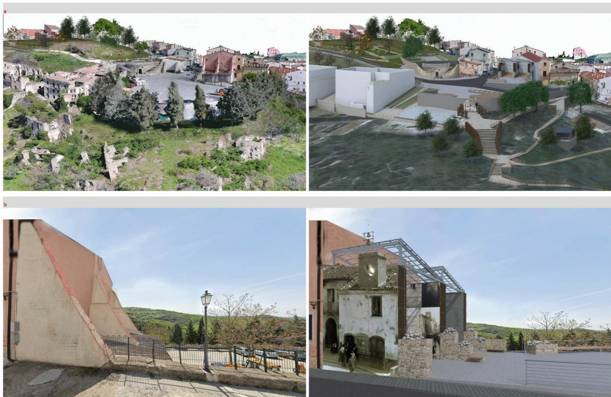
Figure 5b. Via San Rocco's comparison: a. ante-post aerial view; b. ante-post Old Town Hall memory (Source: L.a.co.s.t.a. Laboratory, 2025)
