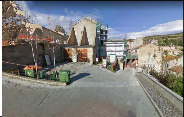
Figure 5a. Via San Rocco: present condition (Source: L.a.co.s.t.a. Laboratory, 2025)
